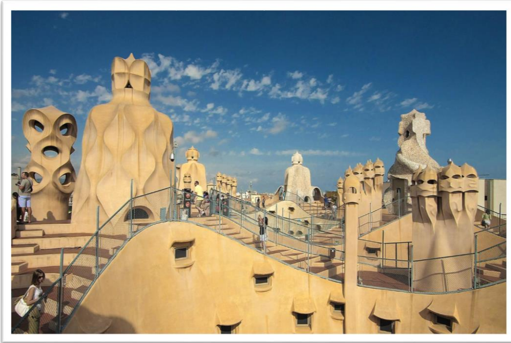
Picture 5 La Pedrera's roof terrace
